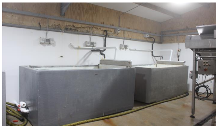
Figure 10: Basic shellfish depuration unit
