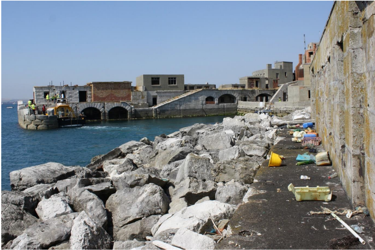
Picture: Washed up litter at Fort Head prior to clean up
